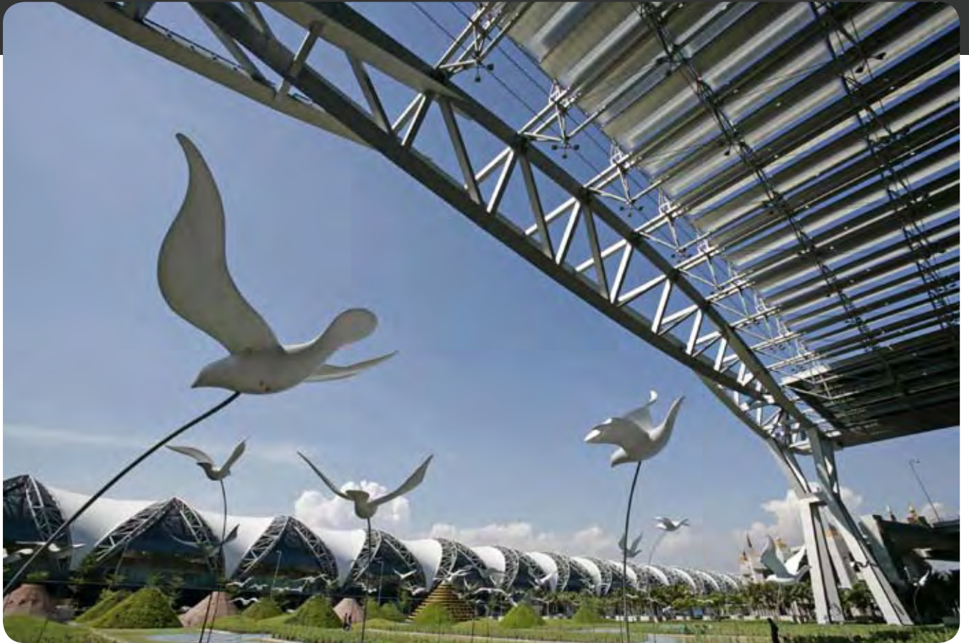
1. STRUCTURAL RIGGING FOR THE SUVARNABHUMI AIRPORT BANGKOK. TENS OF THOUSANDS SWAGED ENDS WAS MADE FOR THIS PROJECT BY A SEVERAL OF OUR CUSTOMERS.
